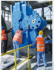
Traditional pinion/girth gear drive with grease spray lubrication.
